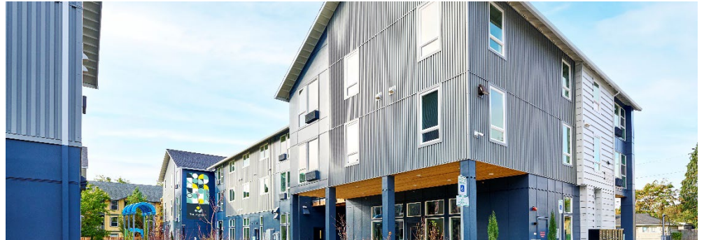
Photo courtesy of Home First
