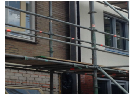
New exterior wall assembly seen over the existing wall
