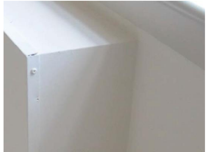
A/C Sleeve Sealed to Drywall
