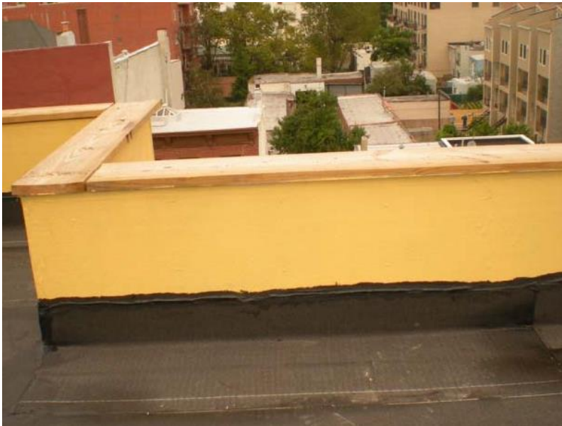
Transition Between Wall and Roof Barrier
